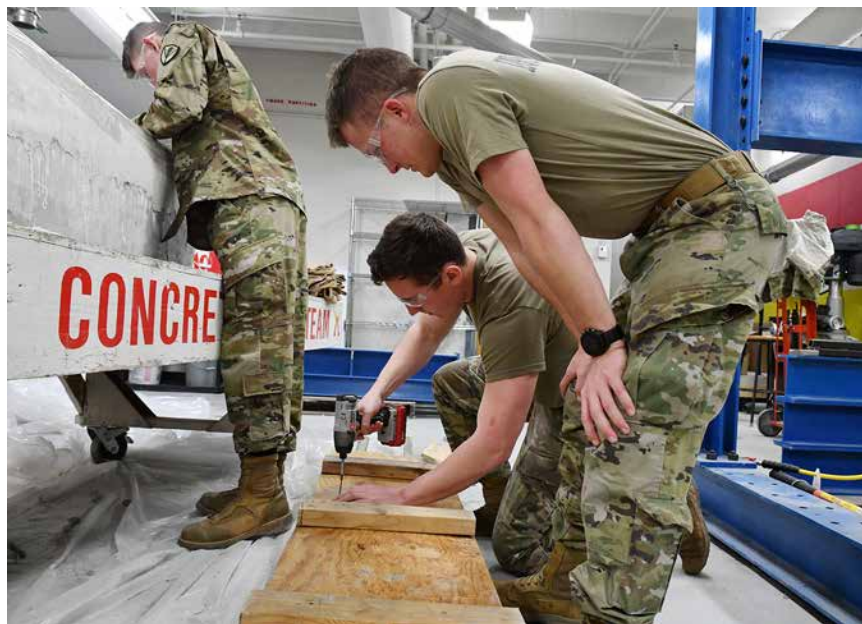
Garret Shultz '20 watches while Jim Tulsiek '20 drills into a wooden form prior to pouring concrete in the civil engineering lab.—VMI Photo by Kelly Nye.
