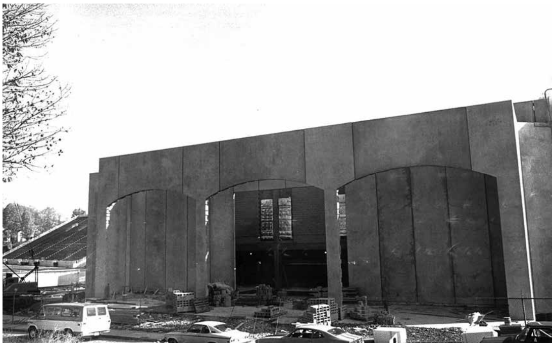
Cameron Hall during its construction in 1980.—Photo courtesy of VMI Athletics.
