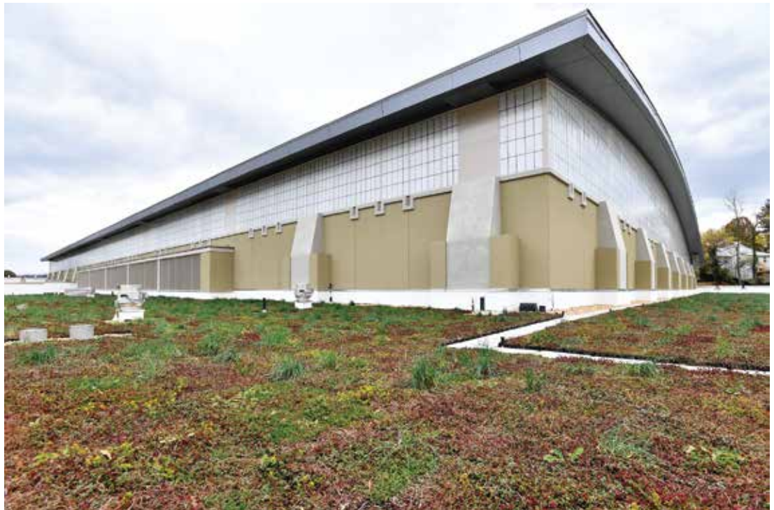
Low maintenance plants on the Corps Physical Training Facility's green roof slow storm water runoff and help insulate the facility. – VMI Photo by John Robertson IV.
