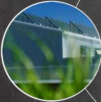
Solar Hot Water
