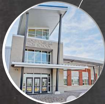
Kellam HS LEED Gold Pending
